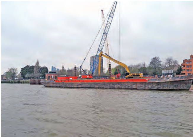
Spoil removal barge at King Edward Memorial Park Foreshore
